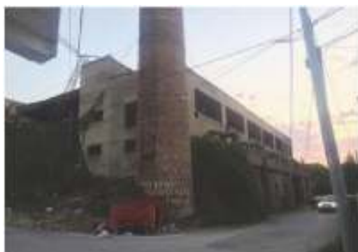
Picture 7 - Photo of site 2/3
