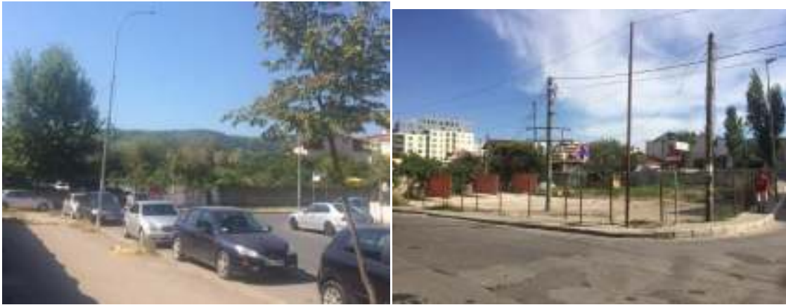
Picture 9 Photo of the site 5/1
