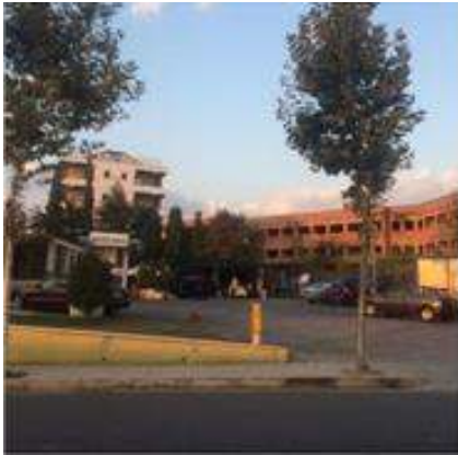
Picture 8 Photo of site 2/6
