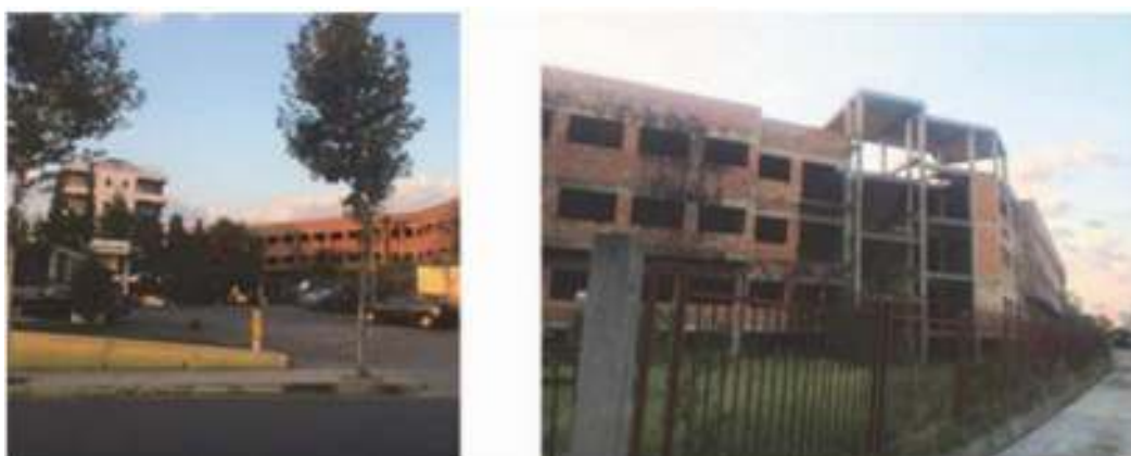
Picture 9 – Photo of the site 2/6
