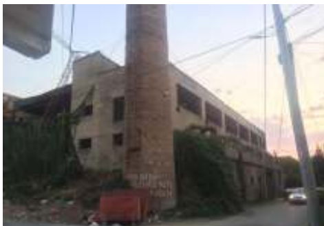
Picture 12 Photo of site 2/3
