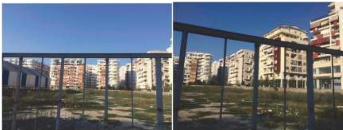
Picture 13 – Photo of site 6/3
